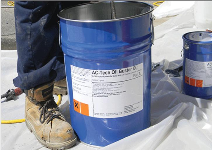
The OBS-C is mixed, spread via a notched squeegee, and back-rolled to ensure even, consistent coverage. After 15 minutes, the OBS-C receives a silica sand broadcast to prevent possible amine blush and delamination of subsequent coatings.
