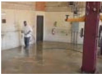
Once oil removal is complete, the entire area is rinsed with a pressure washer using hot water. All excess water should be vacuumed into a suitable containment receptacle and disposed of properly. Water must not remain puddled on the surface of the concrete. The coating process should begin immediately after final rinse.
