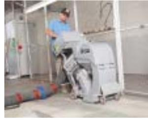
Prior to applying the OBS system, the concrete must be sound, solid and free of all prior flooring materials, coatings underlayments, adhesives and any material that may act as a bond-breaker. The concrete must be edge-ground and shot-blasted to a CSP of 4 in order to allow for rapid and thorough penetration of the OBS-D.
