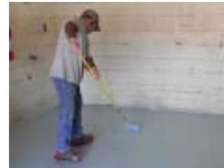
OBS-C is mixed per the technical data sheet's instructions and then poured directly onto the newly cleaned, damp concrete substrate. The material is then evenly spread using a notched (16 mils) or flat squeegee and back-rolled with a suitable 3/8" short nap roller until a uniform thickness is achieved.
