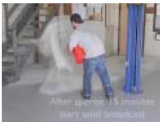
~About 15 minutes after OBS-C application, the fresh coating is broadcast with 50 - 60 mesh washed & dried silica sand to rejection. Once broadcast, the material is allowed to cure for 12 hours, depending on ambient temperature and humidity. After the material has finished curing to accept foot traffic, all excess sand is removed via broom or vacuum.
