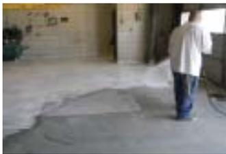
Once the concrete is properly prepared, the surface is then treated with the OBS-D. Using a foaming gun attachment, the OBS-D is mixed with cold water to thoroughly cover the substrate in a "foam carpet". The OBS-D foam is then allowed to soak into the concrete in order to loosen and "float" the contaminants within the slab to the surface.
