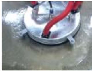
Using a 4000 - 5000 PSI pressure washer, a 180° F water heater and a floor spinner with vacuum attachment, the OBS-D is forced deep into the concrete and the residue and wastewater is then vacuumed into a suitable container. Depending on the level of contamination, steps 3 & 4 may be repeated as necessary to adequately remove contamination.
