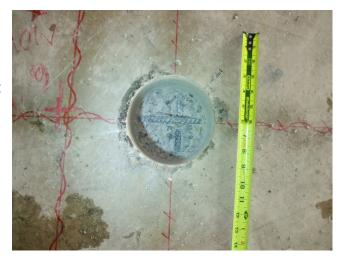
Repairing a core hole with an epoxy type mortar. Fill the bottom of the hole with aggregate stone and/or sand. Be mindful of the surface traffic load and use the appropriate type of filler material.
