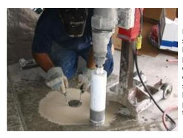
Removing the "short core" after drilling with two screwdrivers. Gently rock the two screwdrivers back and forth in the saw-kerf and the core will pop out for removal. Again, note the mess created on the floor due to the wet drilling. The depth of the core being taken in this photo is shown on the core drill bit where the white paint has been worn off. There is no need to penetrate the entire thickness of the slab unless there is specific reason to do so.
