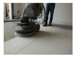
which the concrete surface is prepared that is of utmost importance. Shotblasting tends to give a very good profile or anchor pattern in a controllable, consistent dust-free delivery. Grinding tends to be more inconsistent especially in delivering a constant CSP value of a CSP-3/4 and there is a tendency to impact dust into the concrete surface.
